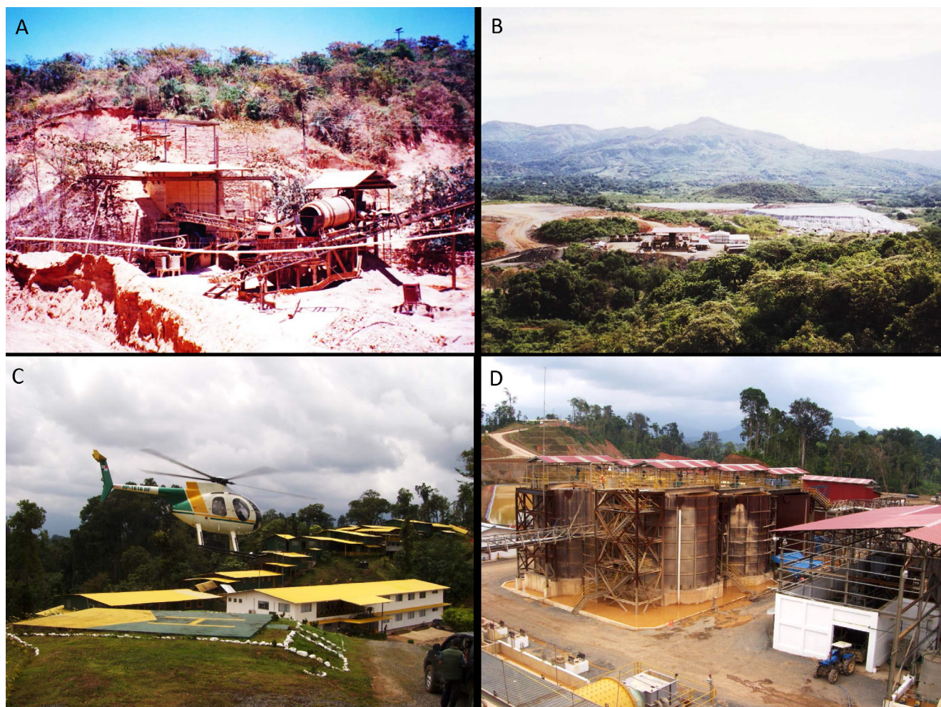
Figure 21 Gold mining in the 1990s to 2010s. A) The crusher and ball mills which fed a 200 tpd carbon-in-pulp (CIP) plant at the Remance gold mine in March 1994. It operated from 1990-1998, the first gold mine in Panama in 50 years. March 1994. B) The heap leach pad and gold recovery plant at the Santa Rosa gold mine, June 1997. It was mined from 1995-1999. C) The Molejon mine camp and office with a Hughes 500 helicopter, March 2009. Gold was mined from 2009-2014. D) The gold CIP leach tanks with 2,200 tpd capacity at the Molejon processing plant, March 2009. (Photographs by Stewart Redwood).
