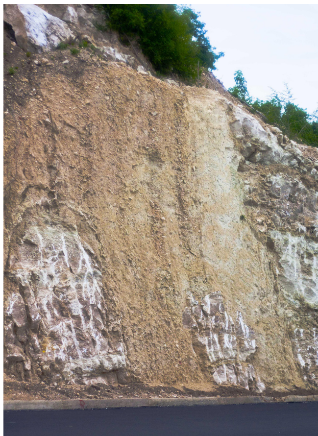
Figure 4 Blocks of massive GM caught up in poorly bedded argillite, part of the same outcrop as in Figure 3 and about 50 m east of that outcrop. Note distinctive tooth marks of the excavating equipment that identifies soft, ductile gypsum and can be used for a virtual field trip along Highway 186 in Google Earth “Street View.”
